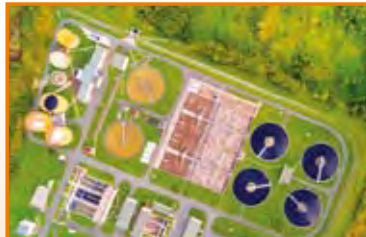
Sewage treatment plants
